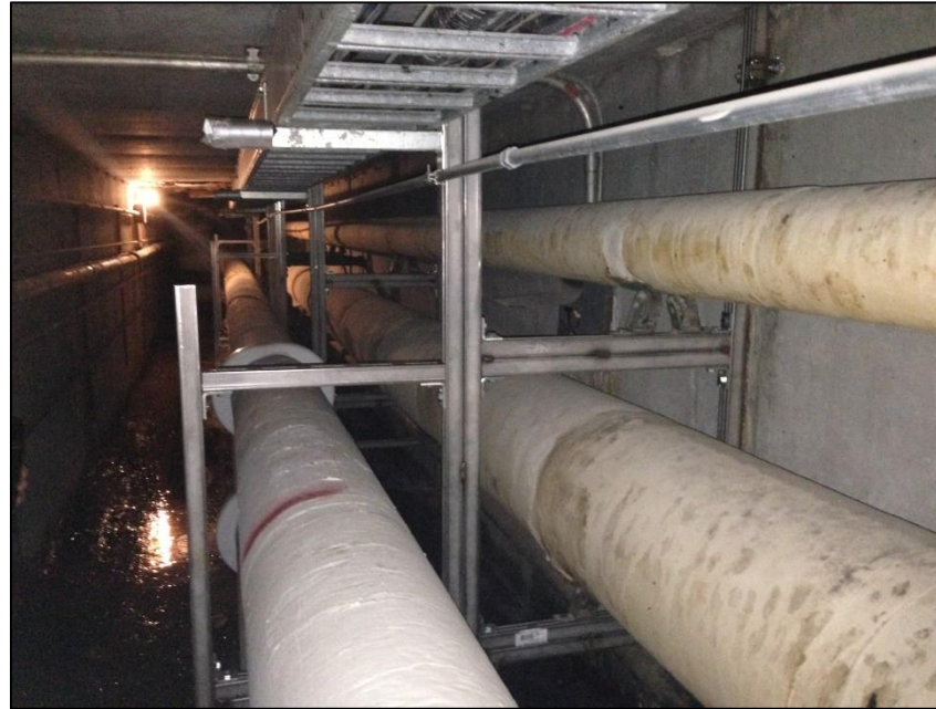
Water is getting through fissures and flooding the tunnels.
