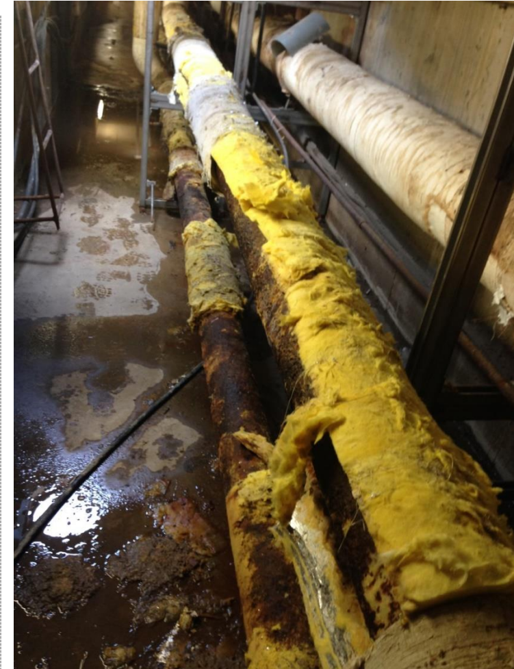
When trench drains collect debris, tunnels below fill with water
